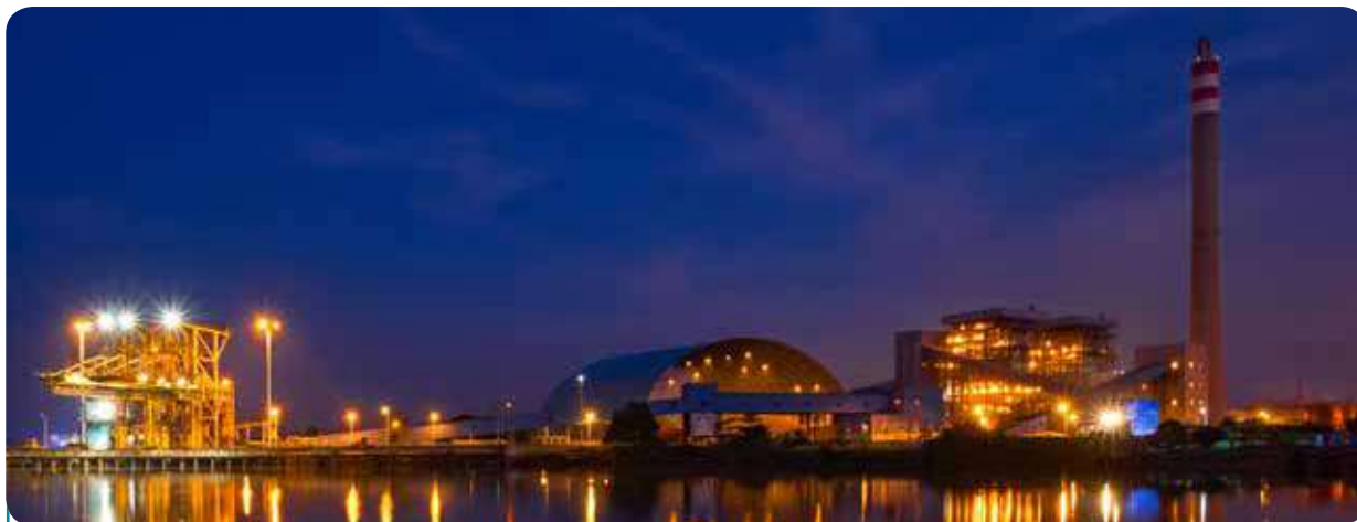
PLTU Tenayan Tenayan CFPP
