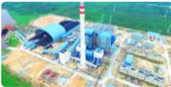
PLTU Tenayan 2 X 110 MW Tenayan CFPP 2 X 110 MW
