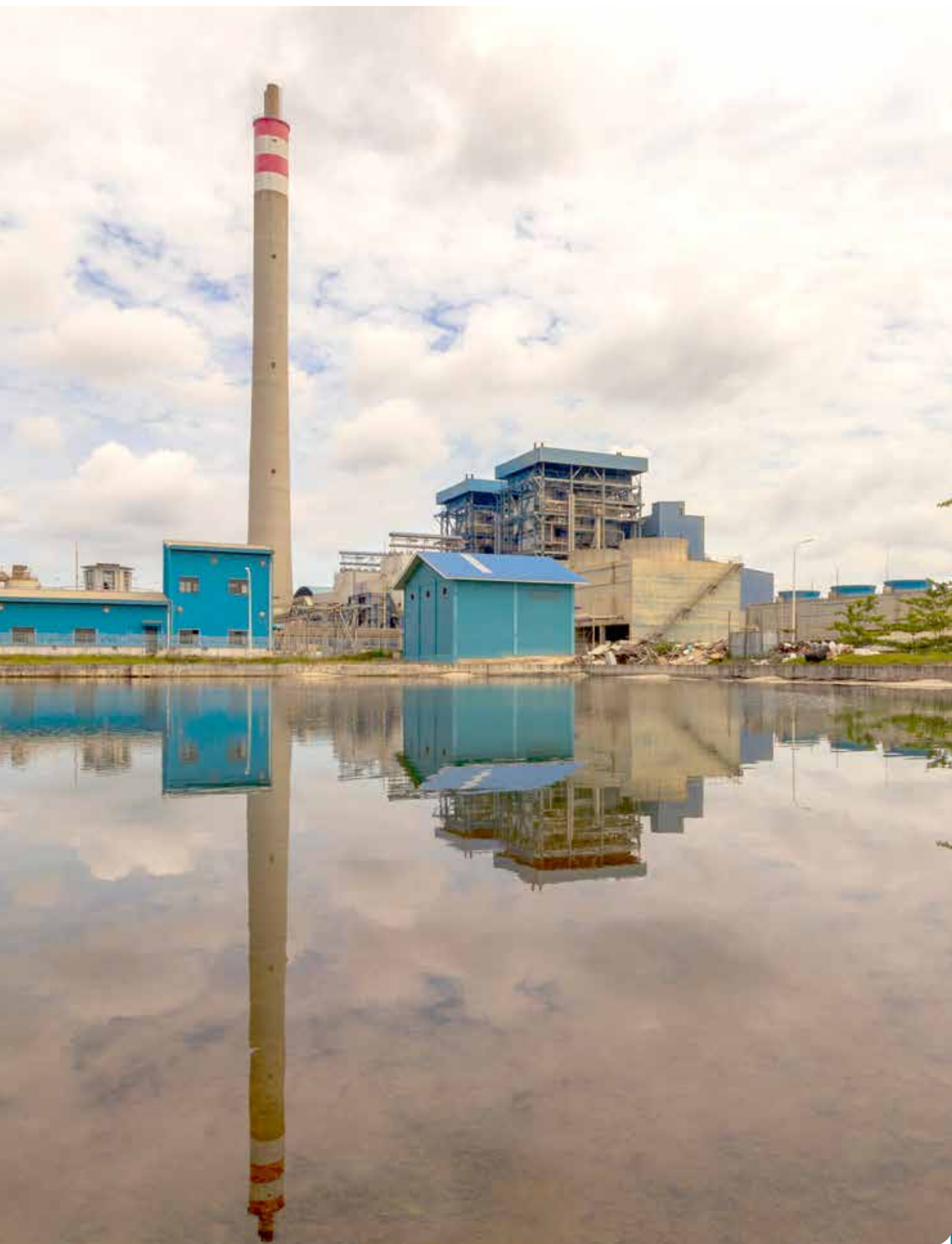
PLTU Tenayan Tenayan CFPP
